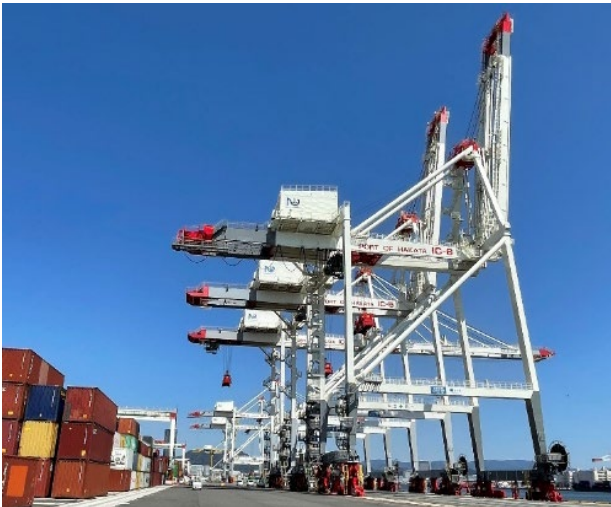
Introduction of 6 STS Cranes with Inverter Control Systems
