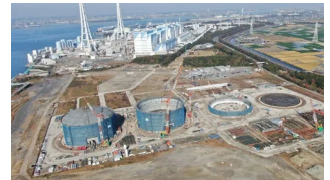
Construction work of ammonia tanks at a thermal power station
