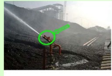
Dust Suppression system, water sprinklers & wind shields
