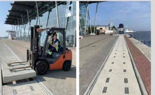
Option 3: Truck with cable reel - cables in duct with removable co
